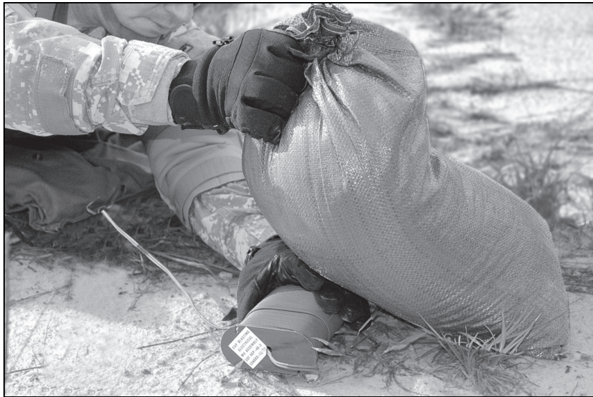
Figure 3-14. Placing the firing wire spool (with the blasting cap) under a sandbag
